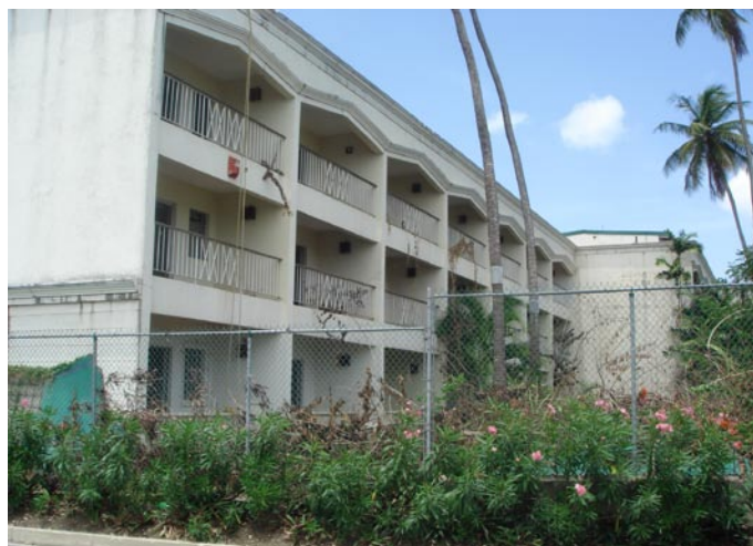
3 View South of existing rear garden
