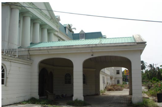
6 View of front entrance structure
