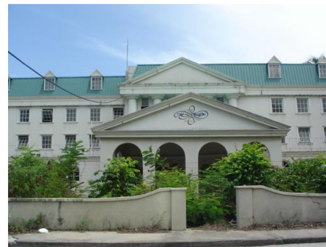
4 View of front entrance
