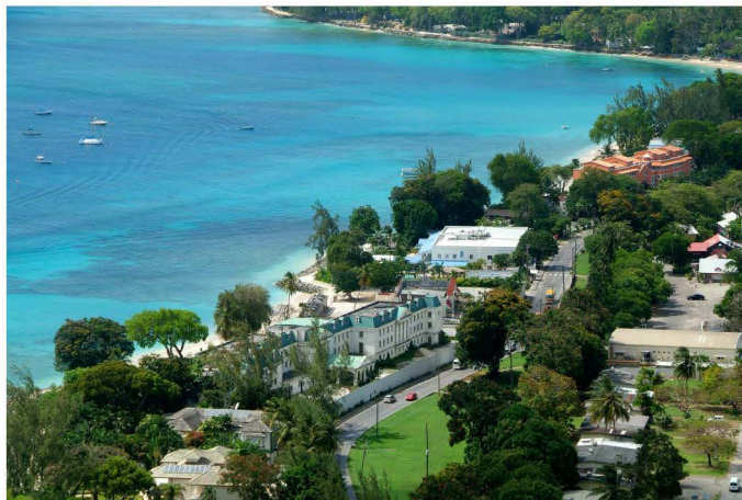
site prior to demolition of previous hotel; source: client
